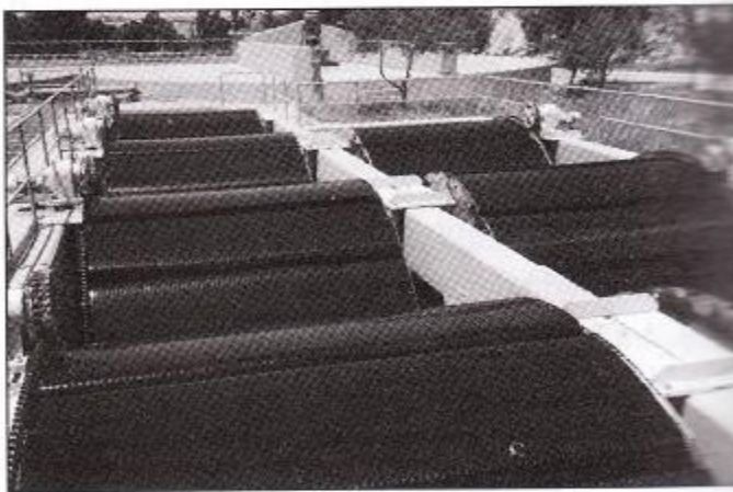
(c) View of RBCs with flow perpendicular to shaft
