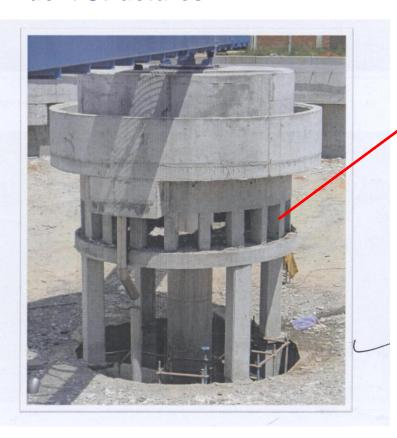
Feeding well diameter 15-20 % tank diameter
