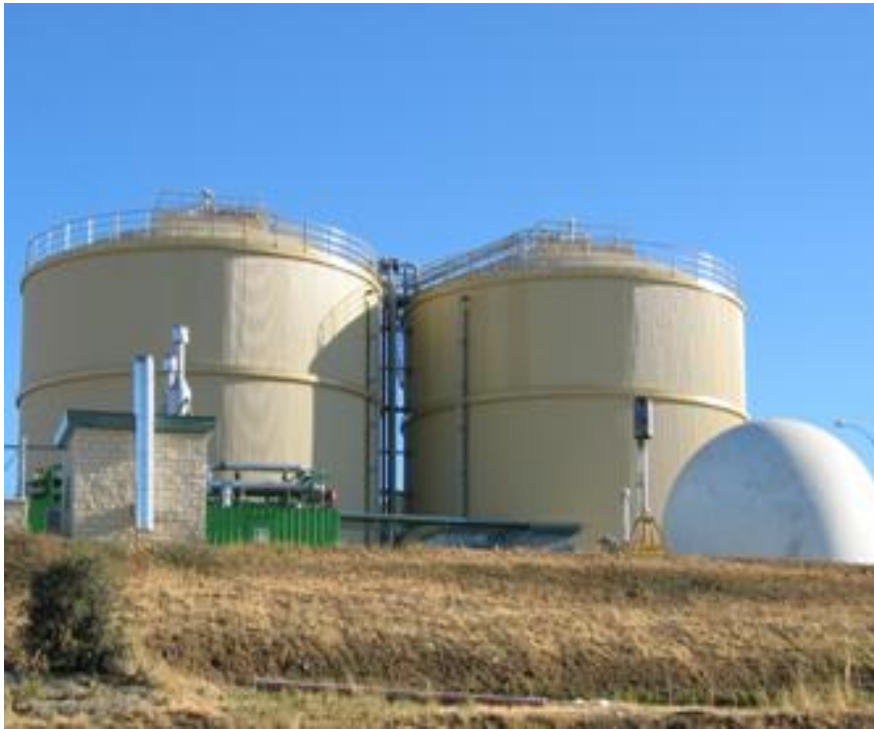
Fixed cover AD with a biogas holder
