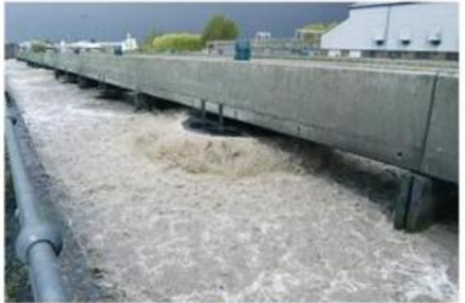
Figure 3.4 Surface aeration in activated sludge treatment plants creates aerosols which contain high amount of microorganisms. This poses a health risk to treatment plant employees and in some cases to neighbors (photo: D. Brdjanovic)
