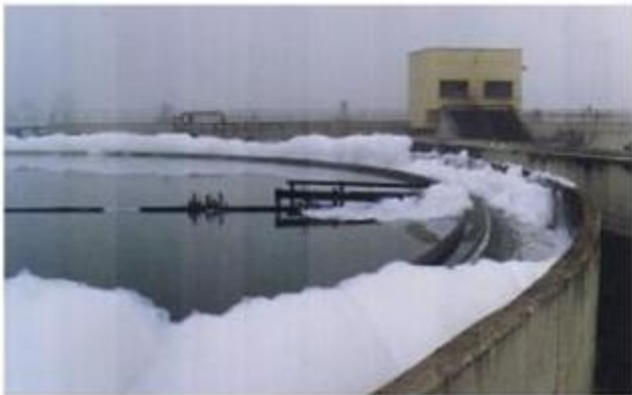
Figure 3-3 Detergents in high concentrations create problems to a wastewater treatment plant operator (photo: M. Henze)
