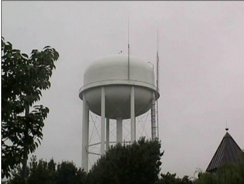
Figure 4. Dome shaped bottom water tower [4].
