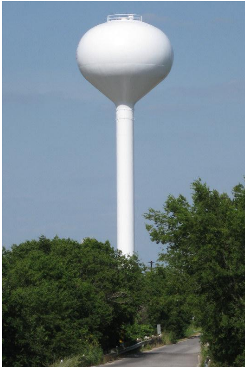
Figure 3. Spherical shaped bottom water tower [3].
