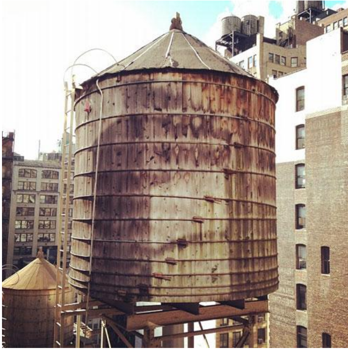
Figure 2. Flat bottom shaped water tower [2].
